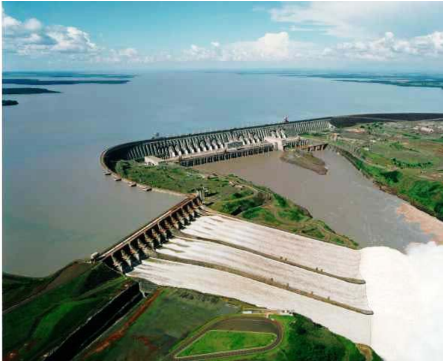
Itaipú dam (BR-PY)
